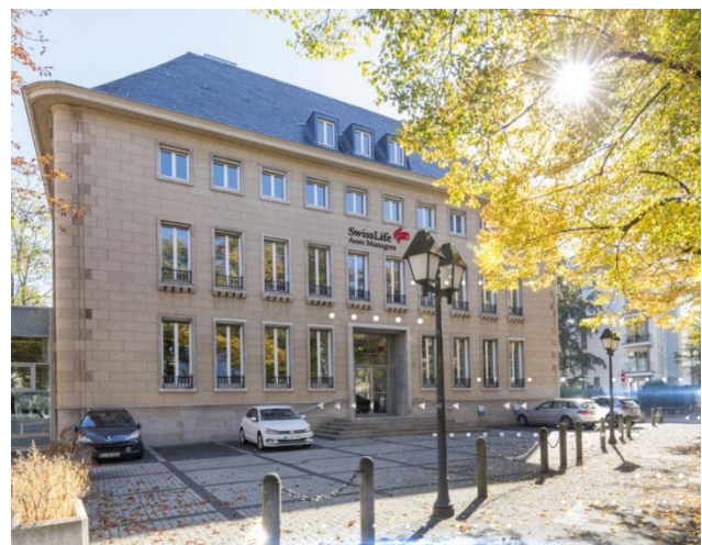
The listed building at Clever Strasse 36 © Swiss Life Asset Managers
