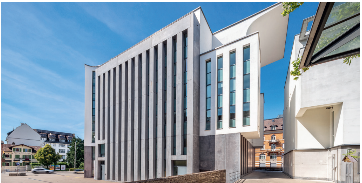
The white striped building is at the head of the former warehouse district, now a commercial area. Source: Fotowerder
