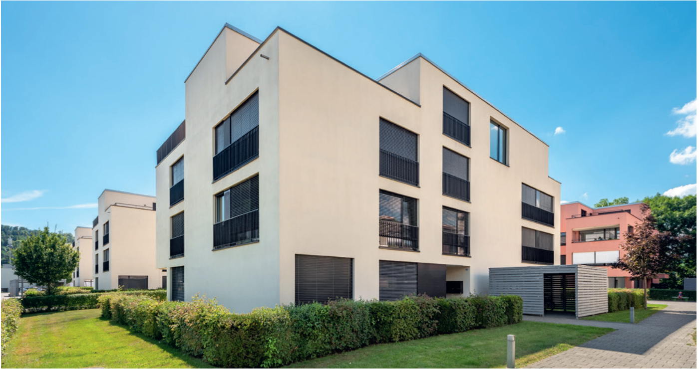
The Minergie-standard buildings are heated with a geothermal heat pump. Source: Fotowerder
