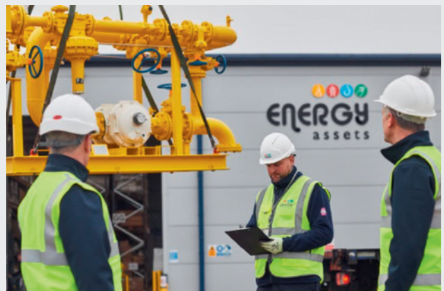
Unloading distribution infrastructure at EAG. Source: Energy Assets Group
