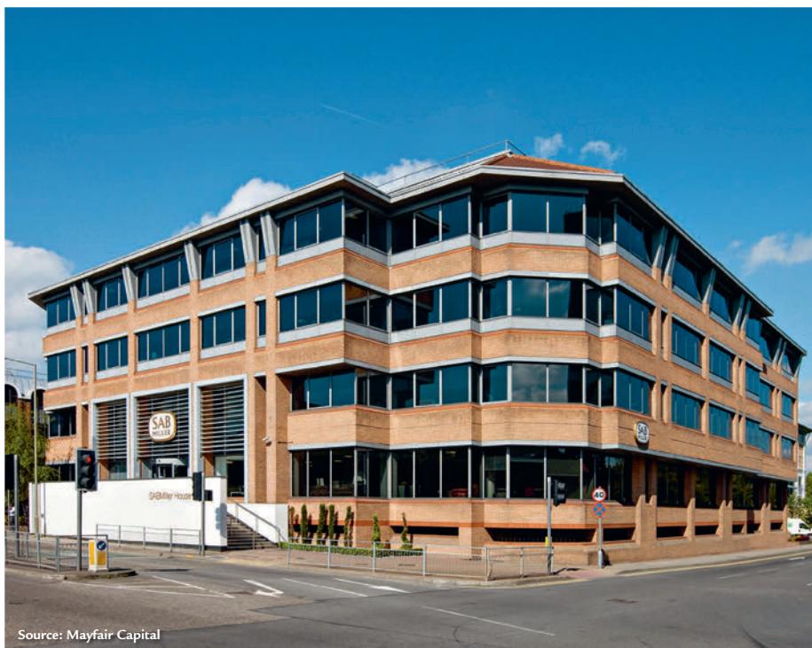
AB InBev House, Woking. This strong thematic purchase by Mayfair Capital provides the potential to create a mix of uses within this building, which itself is in a mixed-use town centre
