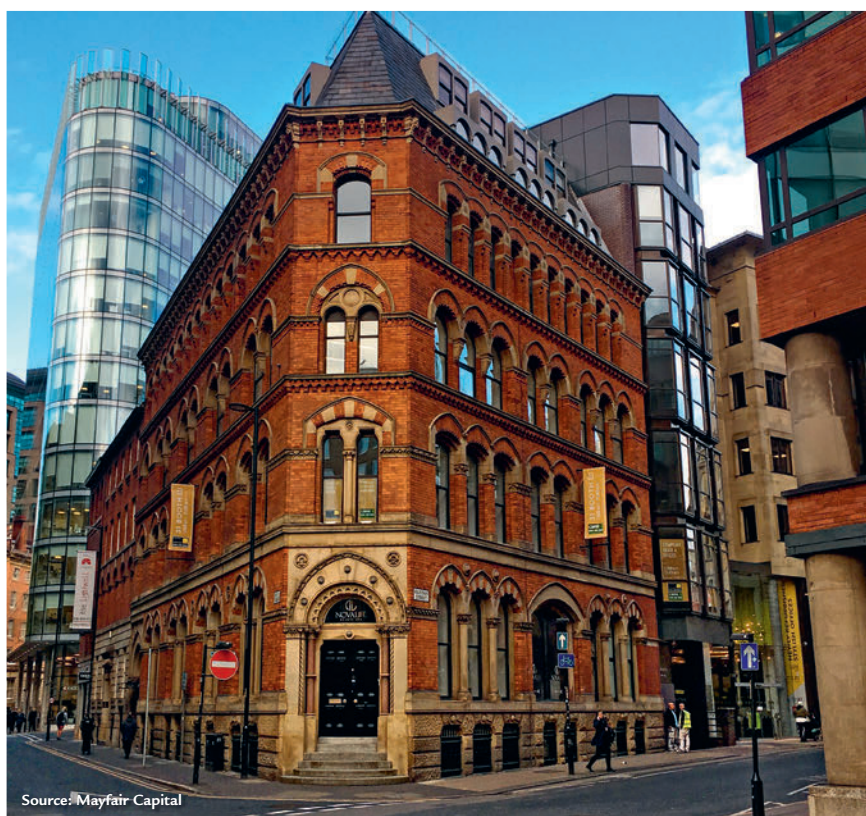
31 Booth Street, Manchester. This recent office acquisition by Mayfair Capital is situated in a vibrant, growing city with opportunities to live, work and play within walking distance
